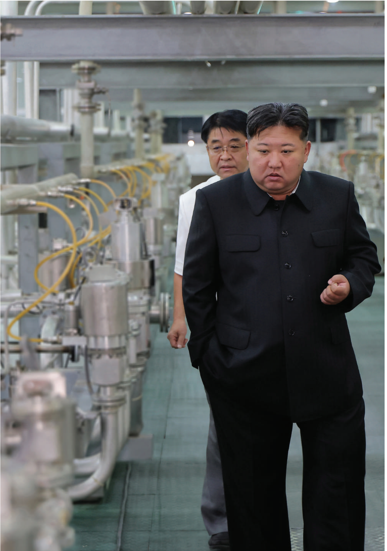
On 13 September 2024, North Korea for the first time publicly announced the existence of its facility for producing highly enriched uranium (HEU), a key component in nuclear weapons. The Korean Central News Agency (KCNA) released photos of North Korean leader Kim Jong Un touring a room filled with centrifuges and reported that the visit was part of his inspection of the country's nuclear weapons research and weapons-grade nuclear material production capabilities. (Photo by EPA/KCNA/NTB)
