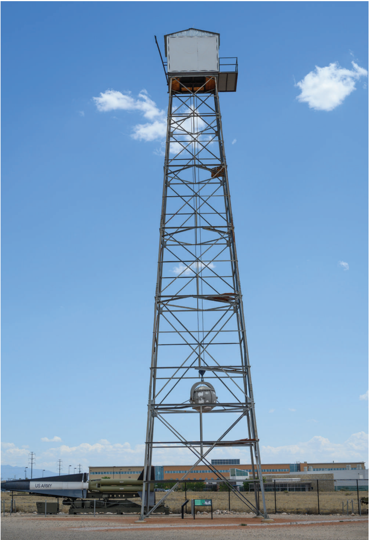
A replica of 'Gadget', the first atomic device tested, hung from a replica of the 100-foot steel tower that was used during the test at the Trinity Site at White Sands Missile Range, is displayed at the National Museum of Nuclear Science & History in Albuquerque, New Mexico. (Photo by Sam Wasson/Sipa USA/NTB)
